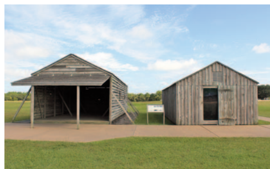
Hangar and living quarters
